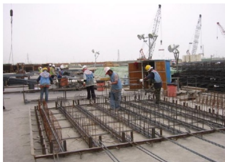
(a) Assembly of reinforcement of waffle slabs for one direction
