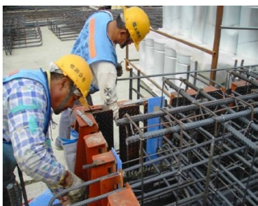
(a) Location of the reinforcement cage
