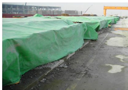
(b) Steam curing of the waffle slabs
