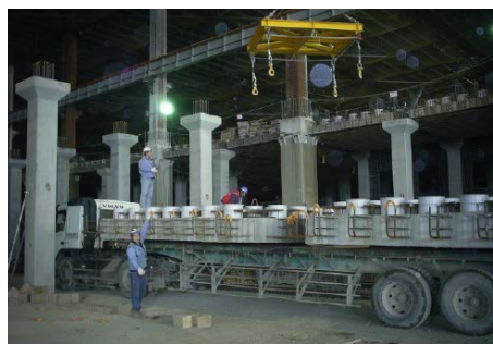
(b) Hoist the precast waffle slabs by overhead cranes
