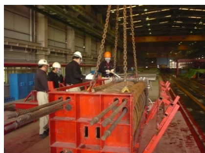
(d) Use templates at both ends of the cages to position the main bars.
