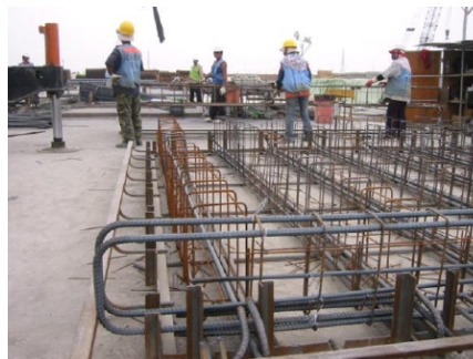
(b) Assembly of reinforcement of waffle slabs for another direction
