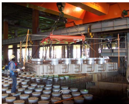
(c) Position the semi-precast slabs
